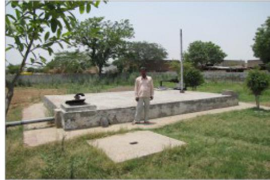
**Figure 5.** Sump of 50,000 ltrs with Booster pump of PHED, Haryana. Two tube-wells, each of 7.5 HP submersible pumps feed this sump. 35 year old one at 1 km delivers saline water, while 3 yr old pump at 2 km provides fresh drinkable water.
