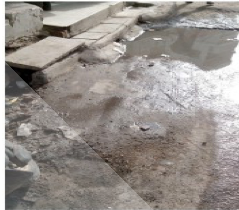
Figure 10. Mixed drain Sewage Overflow Over-road Disposal System.
